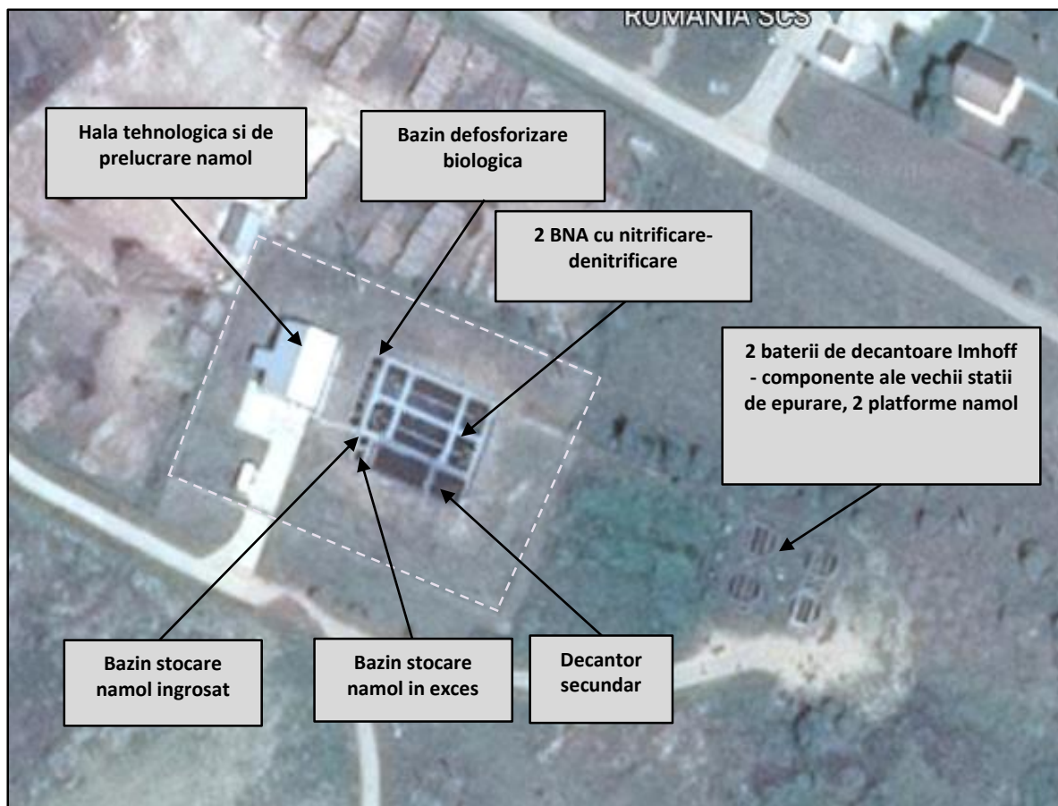
Figura 4.144. Statia de epurare Lipova – situatia existenta (sursa: Internet, Google Earth)
